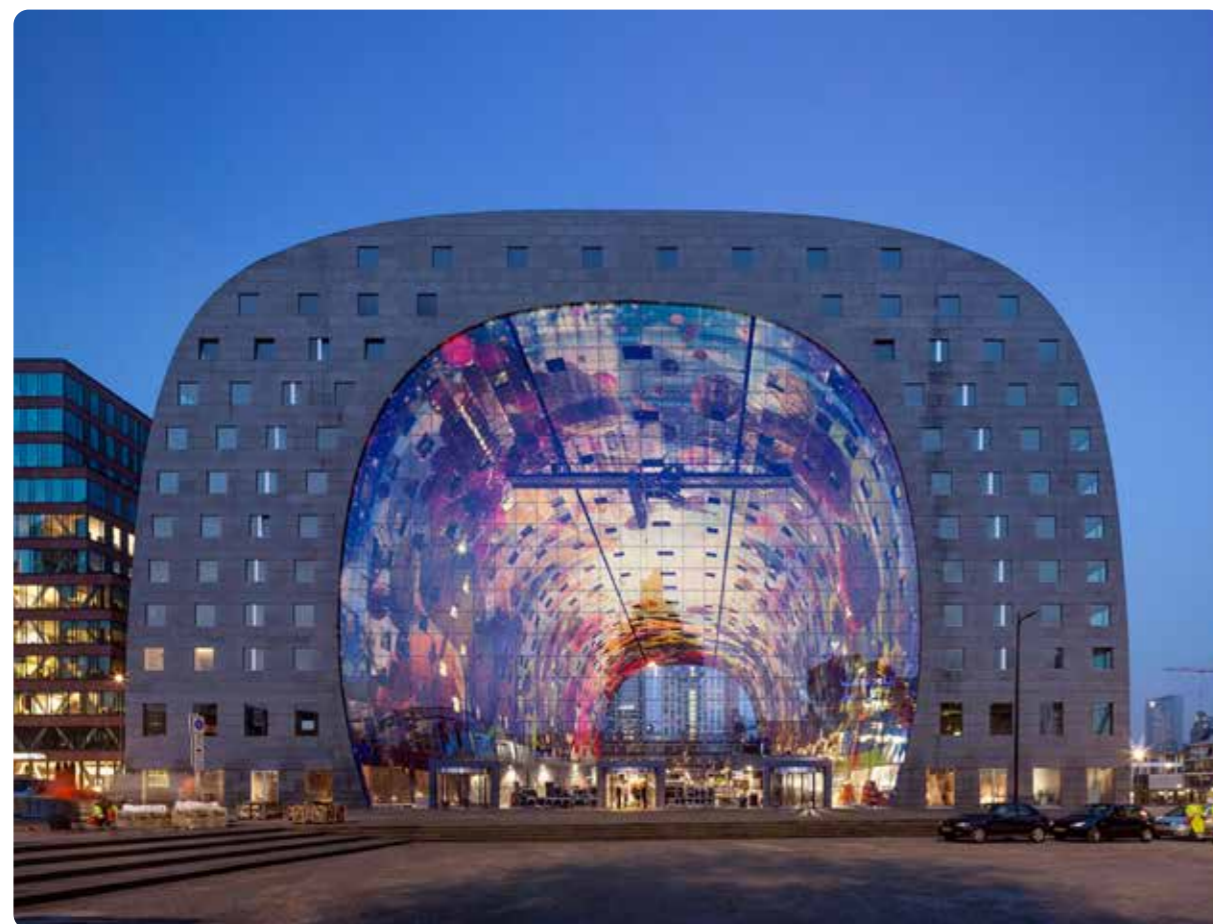
The Markthal, Rotterdam 2014 Rotterdam had a hard time getting people to want to live in the city center. Tourists weren't attracted either. As part of a larger urban renewal effort to make the district attractive again, the Markthal building was erected. Its mix of food market, restaurants, housing and parking created activity from morning to evening. As the building was completed, the tourist numbers in Rotterdam increased from annually 350,000 to 4.5 million people. The building also awakened the desire of Rotterdam citizens to once again live and play in the historic neighborhood. www.markthal.nl
