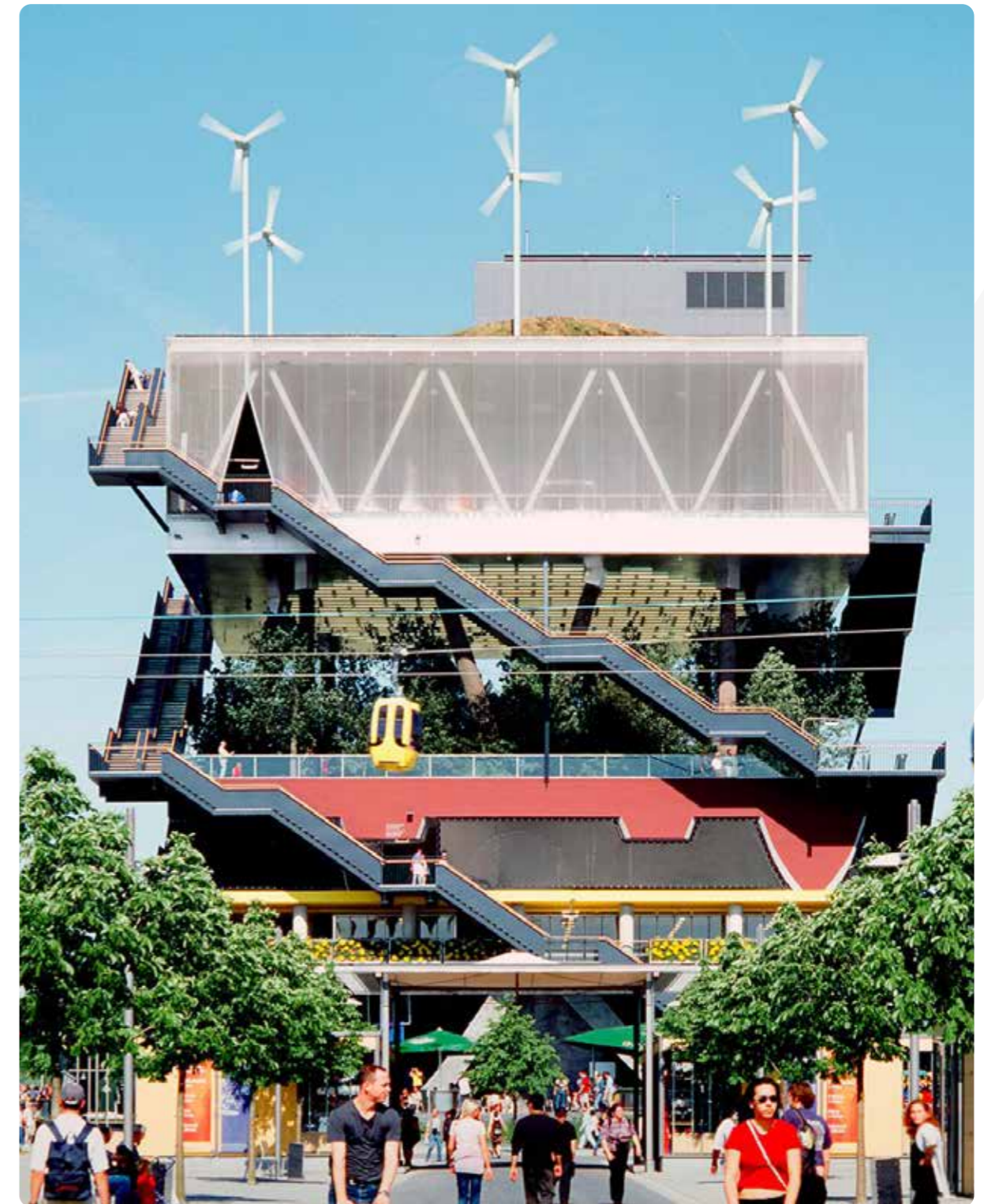
Expo Pavilion 2.0, Hanover, 2020 This was the first time that MVRDV showed that nature could be created artificially within a building. The architecture is also a fine demonstration of the Dutch architectural firm's philosophy about how to densify the city. The theme of the building is "creative space," and it will also serve as a place for co-working. www.mvrdv.nl
